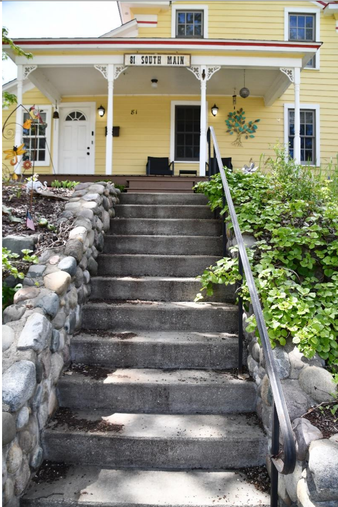
(staircase from the sidewalk – east elevation)
